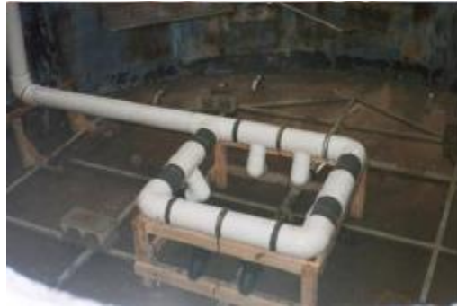
Mixing Nozzles inside the 21 ft diameter tank.
