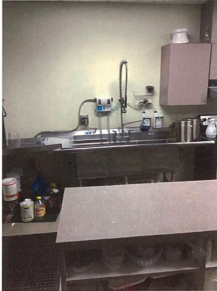
Description: Convention kitchen
